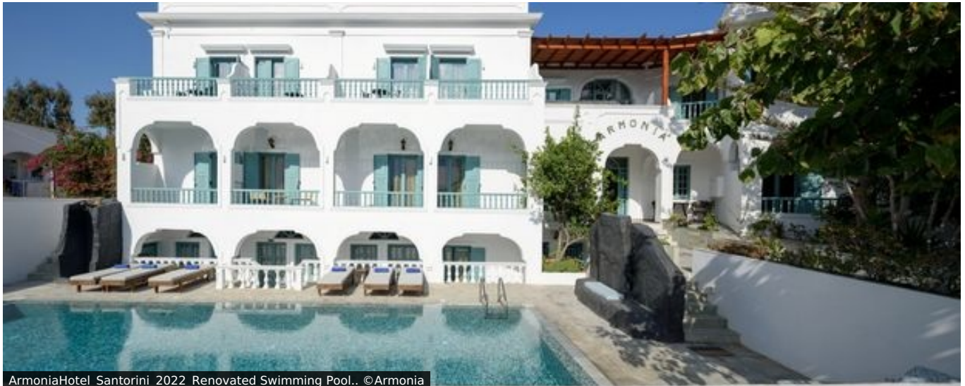
ArmoniaHotel_Santorini_2022_Renovated Swimming Pool.. ©Armonia
